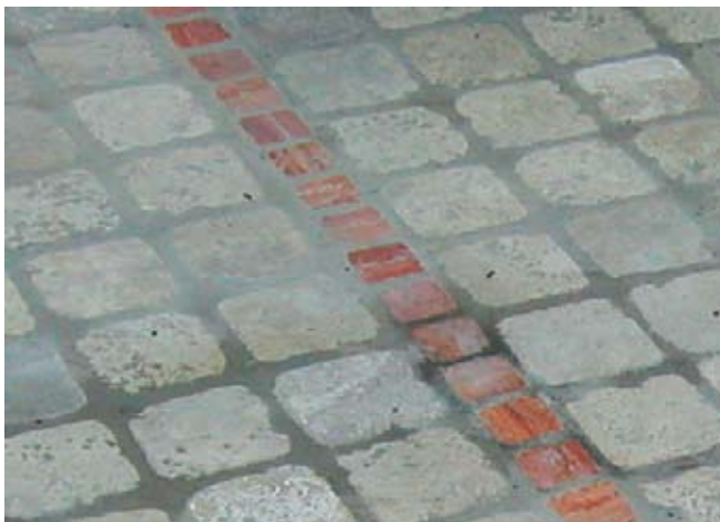
Tumbled marble floor before cleaning.
