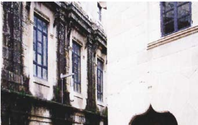
Maintenance was carried out on both these buildings at the same time, but only the one on the right was protected with HYDROREP .
