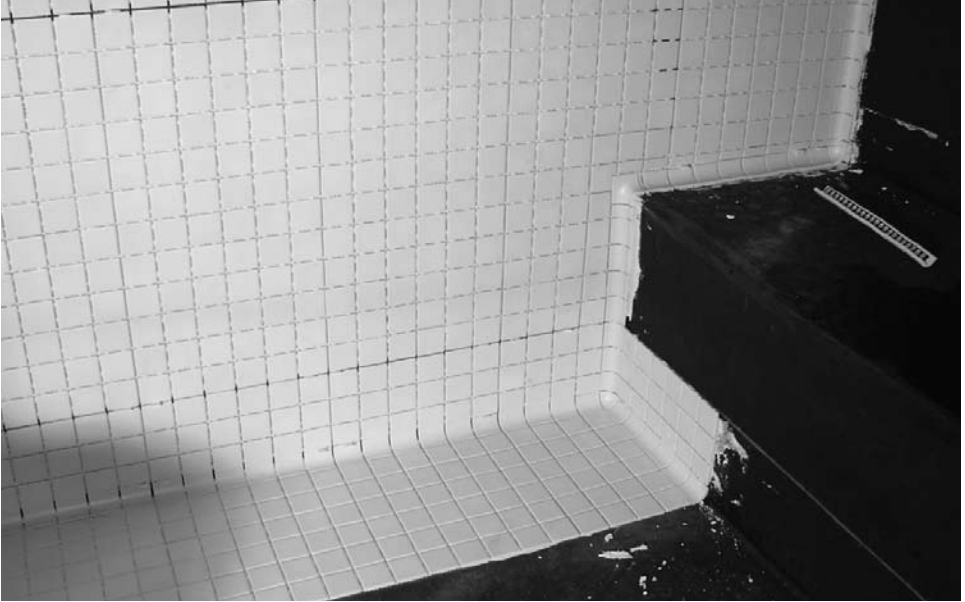
Installation of tile onto LATICRETE 9235 Waterproofing Membrane using LATICRETE 254 Platinum.
