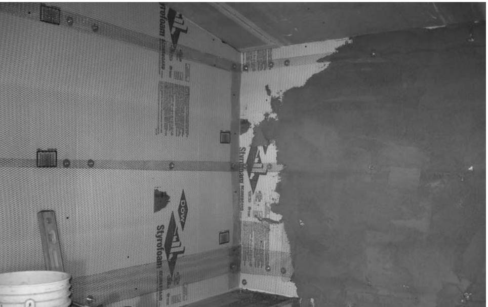
Wall partially finished with scratch coat of LATICRETE® 226 Thick Bed Mortar and LATICRETE 3701 Mortar Admix.
