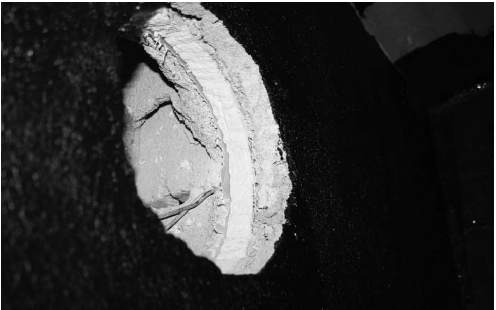
Lighting fixture waterproofing membrane pre-treatment. The vapor retarder, insulation board, mud bed, and LATICRETE 9235 Waterproofing Membrane are all clearly visible.
