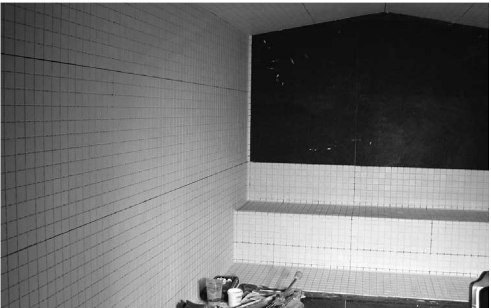
Continuing installation of tile onto all surfaces using LATICRETE 254 Platinum.
