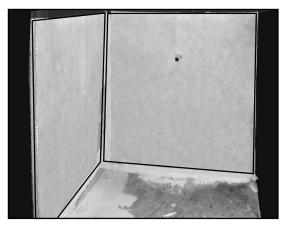
NOTE: Sections of HYDRO BAN® Sheet Membrane may also be shingled (overlapped) during installation without the need for HYDRO BAN Sheet Membrane Sealing Tape. The top section must overlap a minimum of 2" (5cm) onto the bottom section of HYDRO BAN Sheet Membrane.
